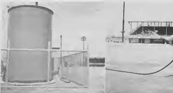
NEW LAGO Sport Park water tank is expected to reduce considerably the chronic dust problem. Tank holds 9000 gallons and can discharge twenty to twenty-five gallons a minute. E tanks a beds completi April 15.
